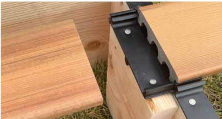
Additional framing may be needed for inline boards (Step-Clips cannot be shared by inline boards).
