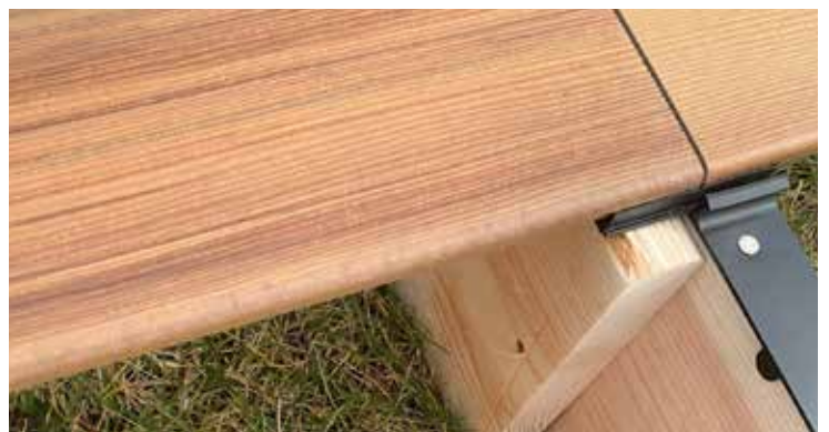
Sister or add framing where butt joints occur then trim a single Step-Clip strip section to accommodate each board and attach separately to the additional framing.
