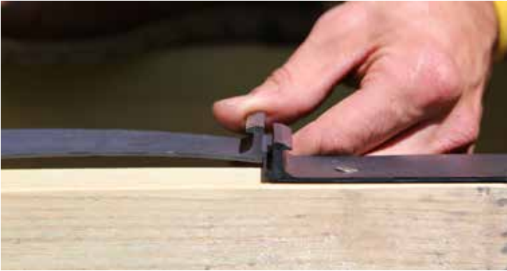
Interlock clip strips along each joist and fasten with roofing nails. Clip strips at opposite end of deck will likely need trimming.
