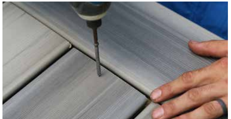
Align and secure interior boards with composite deck screws located at one end of each board (min. of \frac{5}{8} " (16 mm) from board edge).
